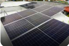
INSTALLATION OF SOLAR PANELS
