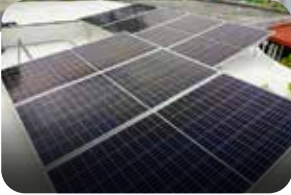
INSTALLATION OF SOLAR PANELS
